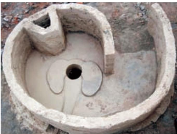
The Elephant Toilet uses just two bags of cement rather than the seven bags that are used for the Blair/VIP Latrine design that the Government of Zimbabwe has selected as its standard technology for rural sanitation projects\*. The cement in the Elephant Toilet is mainly used to mould a reusable slab that sits above the main toilet pit.
