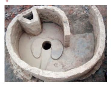
The Elephant Toilet uses just two bags of cement rather than the seven bags that are used for the Blair/VIP Latrine design that the Government of Zimbabwe has selected as its standard technology for rural sanitation projects\*. The cement in the Elephant Toilet is mainly used to mould a reusable slab that sits above the main toilet pit.
